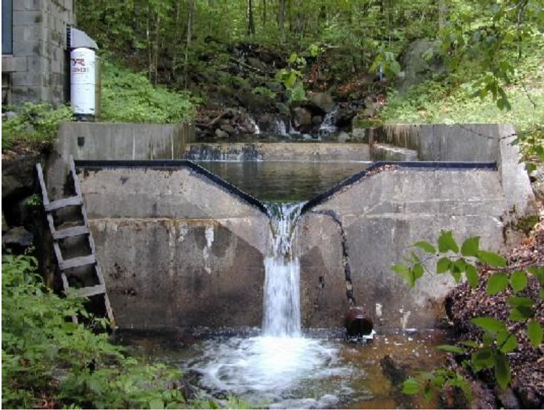
Figure 42. V-notch weir.
