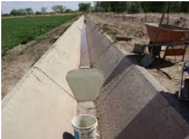
Figure 33. Casting an RBC flume in an existing canal.
