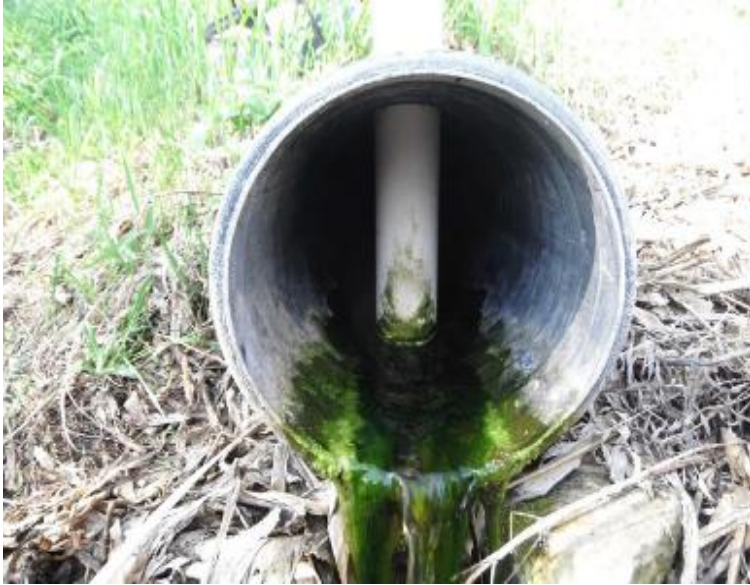
Figure 7. Circular flume in North Dakota used to measure drainage discharge.
