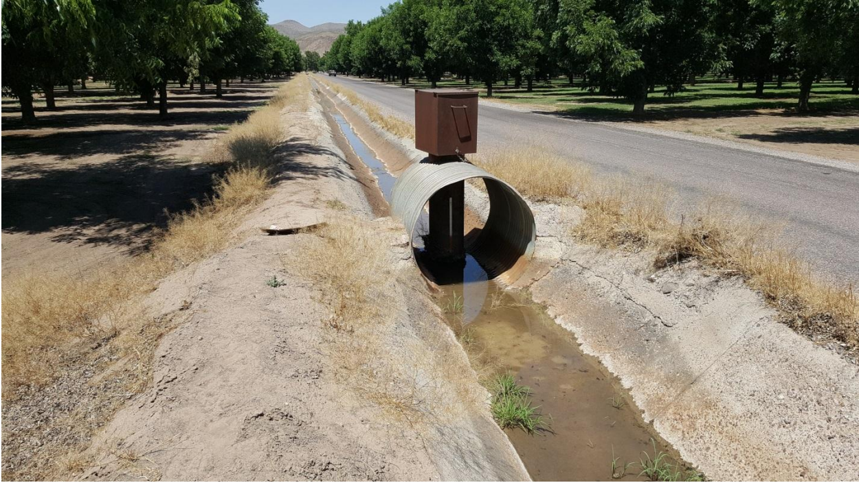
Figure 3. Circular flume in southern New Mexico irrigation canal, located at GPS coordinates: 32.359167, 106.784722.
